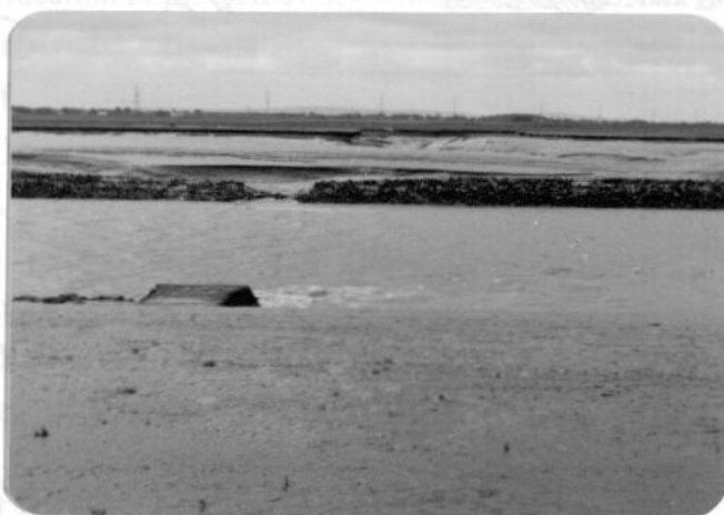
Plate 5 A sewage outfall into the Ribble channel. The habitat in the foreground is muddy sand in the foreground, with a training wall composed of boulders and cobbles on the opposite bank of the channel. [MNCR slide N°: S38.5.3 Dave Mills]
