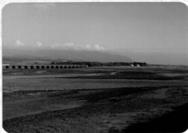
Plate 3 Lower River Esk with the railway viaduct in the background, note the sand and gravel banks within, and adjacent to, the river channel. [MNCR slide N°: S38.GEN.1 Chris Emblow]
