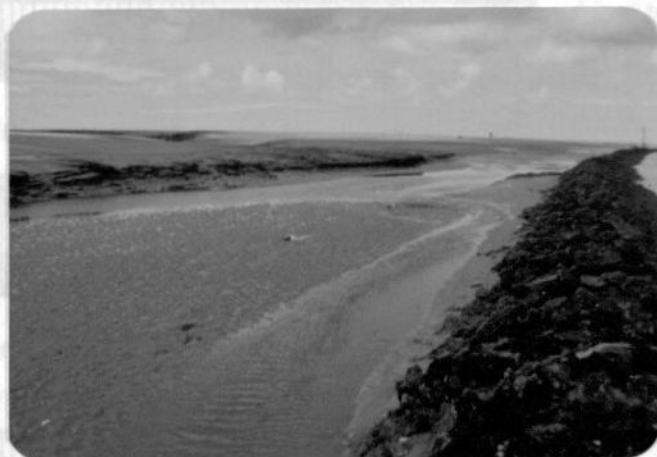
Plate 7 A training wall composed of boulders and cobbles, backed by extensive sediment flats, at the mouth of the Ribble Estuary. [MNCR slide N°: S38.2.2 Roger Covey]
