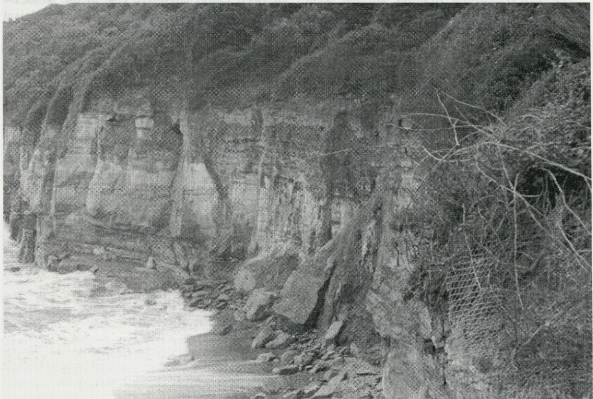
Figure 6.14 Cliff End. The sea is washing beds of the upper Ashdown Formation within which the Isoetites plant fossils are found. The massive sandstones above belong to the Cliff End Sandstone within the Wadhurst Clay Formation. (Photo: D.J. Batten.)
