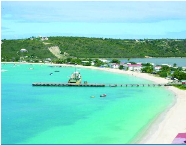
Anguilla Harbour is vulnerable to sea level rise due to its low-lying location. Credit: Anguilla National Trust
