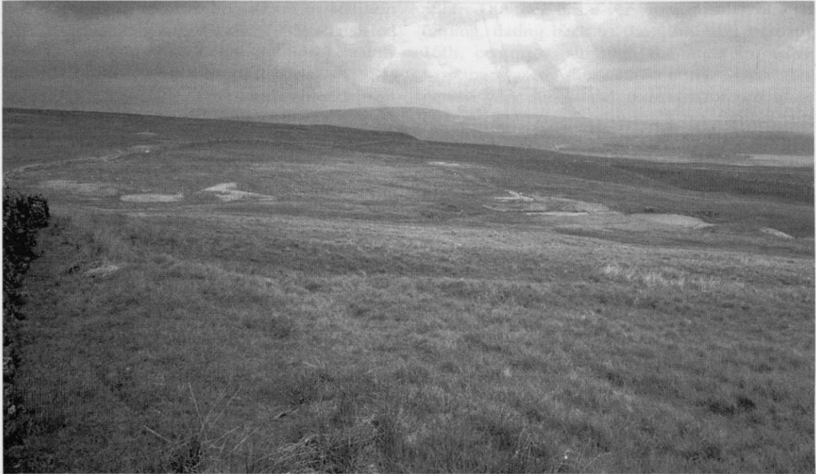
Figure 3.20 Looking west across the site of Pikedaw Calamine and Copper Mines. Spreads of tailings from hand dressing of copper ores are conspicuous. The calamine shaft lies near the centre of the view in the middle distance. (Photo: BGS No. L2755, reproduced by permission of the British Geological Survey, © NERC. All rights reserved. IPR/105-15CX.)
