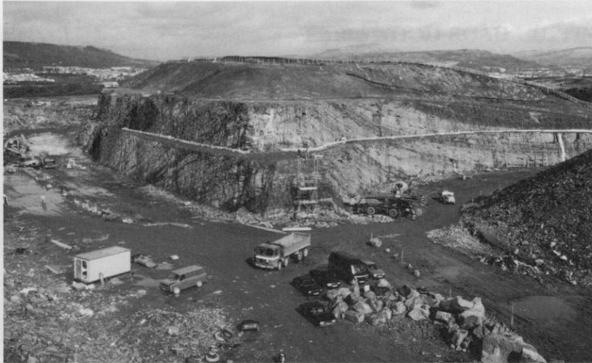
Figure 4.23 Earlswood Roundabout (March 1992): newly created cutting at the cusp between the slip road and main carriageway of the M4 extension between Briton Ferry and Lon Lâs. Excellent dip and strike sections through the Rhondda Member (Pennant Formation) enable detailed sedimentological studies to be conducted in this complex deltaic succession. (Photo: S. Campbell.)
