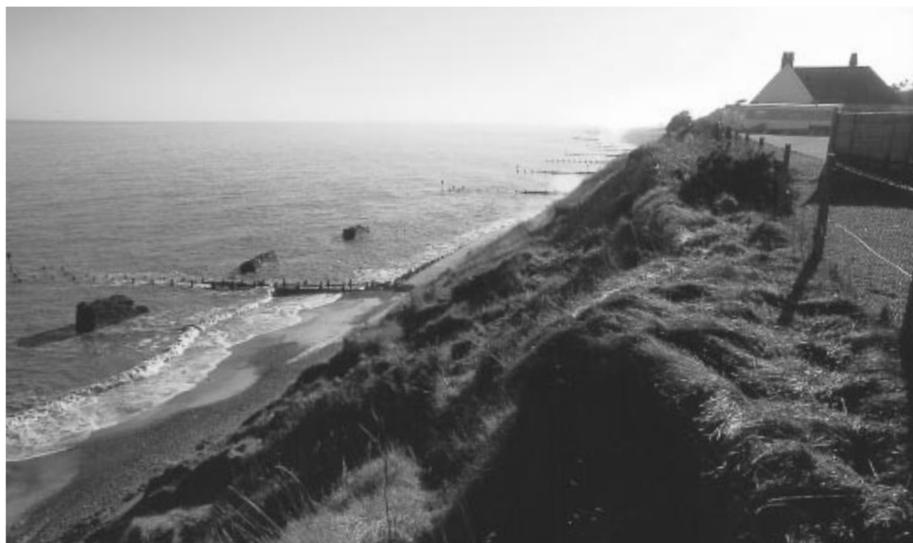
The southward tidal current off the Suffolk coast carries a heavy burden of sand and shingle eroded from the soft cliffs. This house is temporarily protected by the remains of old cliff protection works, which break the power of the waves, and a groin parallel to the cliff, which retains sediment at its foot. Photo: Peter Wakely, English Nature.
