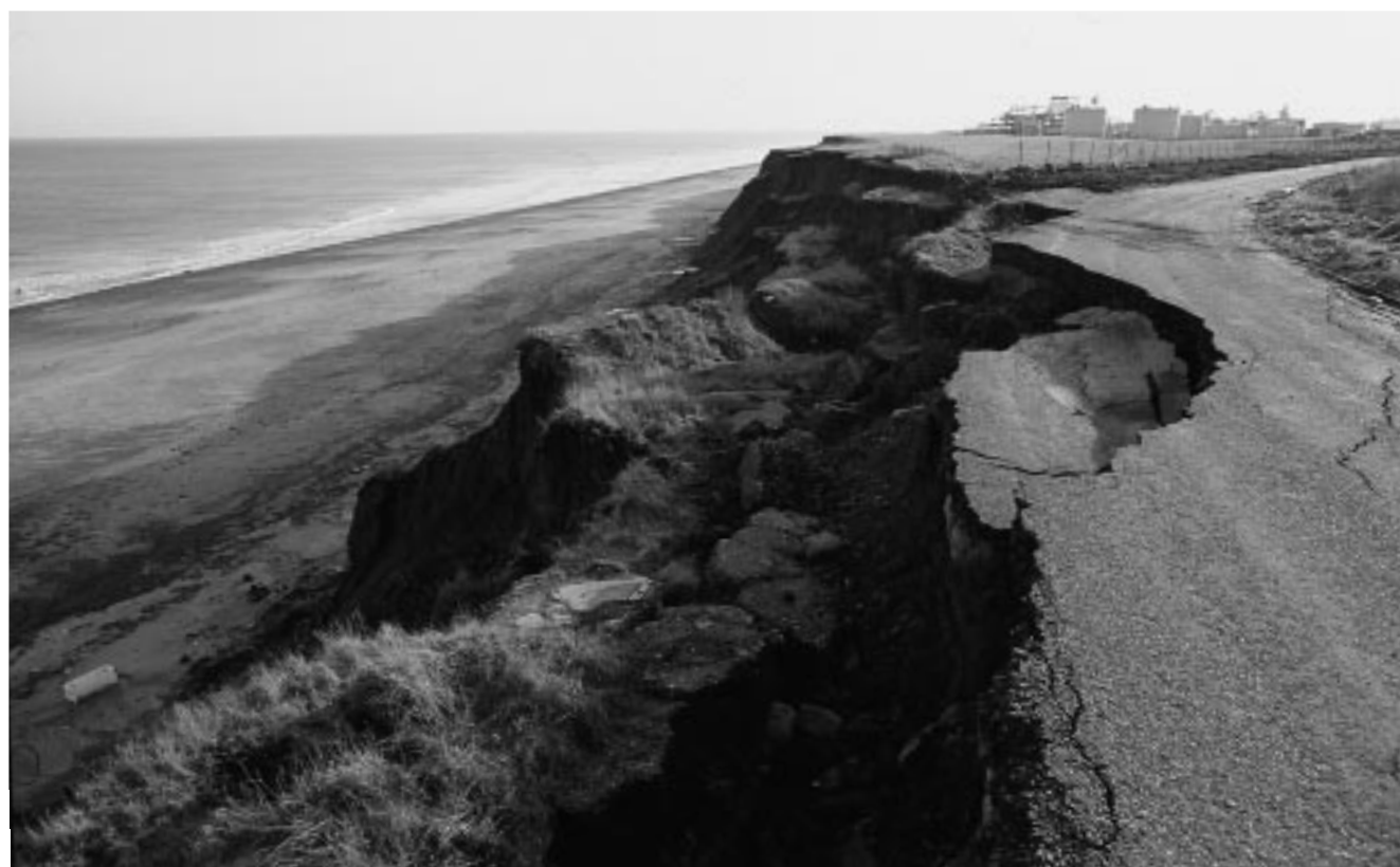
The Holderness coast, North Humberside, is the fastest eroding stretch of coastline in Europe: up to a metre of land is lost every year. Destruction by these powerful natural processes is usually unavoidable for all except high-value installations, or where human lives are at risk. The cliff-top gas terminal at Dimlington is one such priority site. Photo: Peter Wakely, English Nature.
