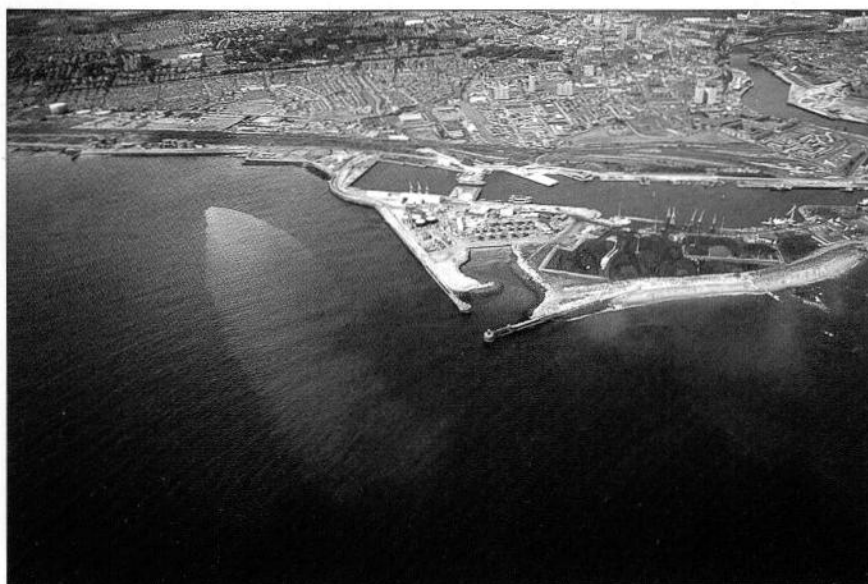
Some of the coastline of Britain has been greatly altered by development, coastal protection and by disposal of wastes; sometimes creating habitats and assemblages of species not found on nearby natural coasts but often destroying irreplaceable natural features: Sunderland Harbour and sea outfall, Tyne & Wear (Rohan Holt/JNCC).
