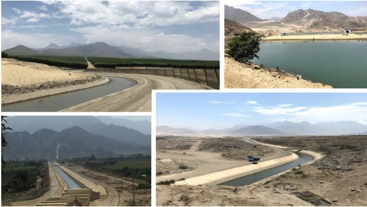
Figure 1. Chavimochic Project connects four river valleys in La Libertad, the Chao, Virú, Moche, and the Chicama, via an irrigation canal. The first two phases of the project are complete, costing US$1.29bn. A third phase is planned, including constructing a 360 million m 3 reservoir in Palo Redondo, a third line of the Virú water pipeline and 113km Moche-Chicama-Urricape water channel.
