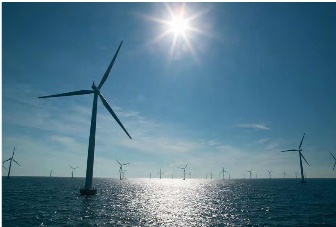
The Nysted Offshore Wind Farm in the Danish part of the Baltic Sea consists of 72 turbines situated c. 11.5 km south of the island of Lolland and covering an area of 24 km 2 . Water depth in the area is 6 - 9.5 m. The windfarm has a total power capacity of 165.6 MW, and is the world's largest offshore wind farm. (Photo provided by Energy E2). Photo: Ib Krag Petersen.
