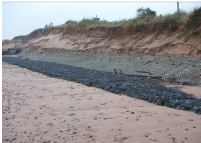
Figure 4. Dune stabilisation, Dawlish Warren NNR. Originally covered by sand, the matting and rocks has subsequently been exposed after erosion by a storm, and may actually now inhibit dune re-establishment. (© Phil Chambers).
